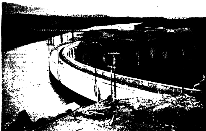
FIG. 145. THE ARAPUNI DAM
